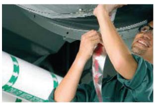
Scotch® Foil Tape 3326, Silver (UPC: 00-051131-85494-9) *Minimize air leaks in HVAC systems by sealing duct joints, insulation and blower compartments.*
